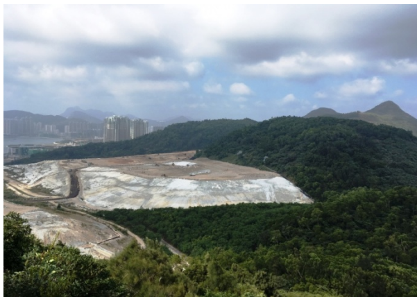
West over the Tseung Kwan O landfill
